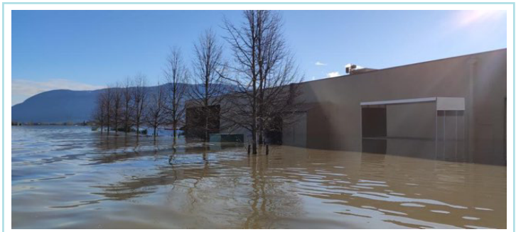
This photo shows how high the water reached in the area.
