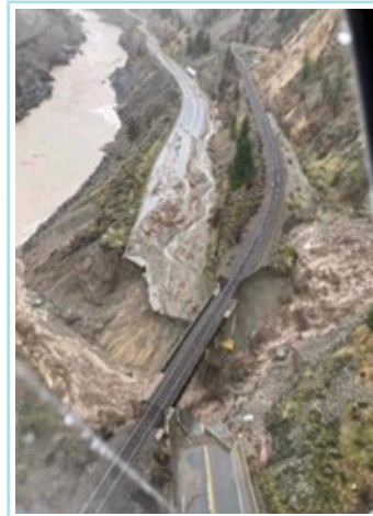
A screenshot of the devastation caused by the flooding in BC.
